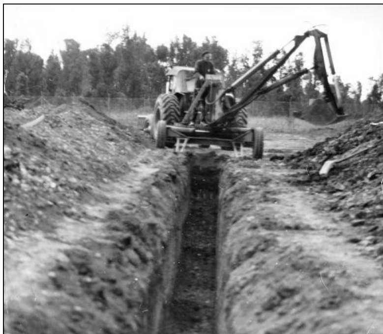
Figure 5. Excavation of trenches at LFBG.
