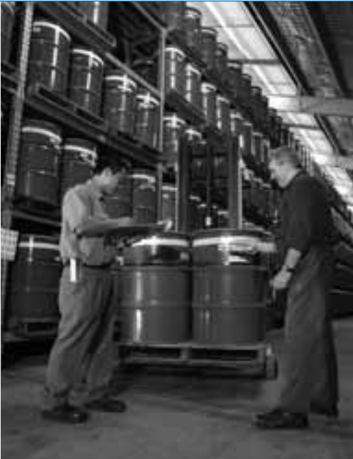
Low-level waste storage facility. Low-level waste contains very small amounts of radioactivity and does not require shielding to protect workers during normal handling or transportation. Ninety-eight per cent of waste produced by ANSTO is low-level waste, comprising paper, plastic, gloves, cloths and filters which contain small amounts of short-lived radioactivity.
