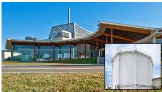
Figure 1: Australia's current research reactor, OPAL, in the background, with the first reactor, HIFAR, in inset.
