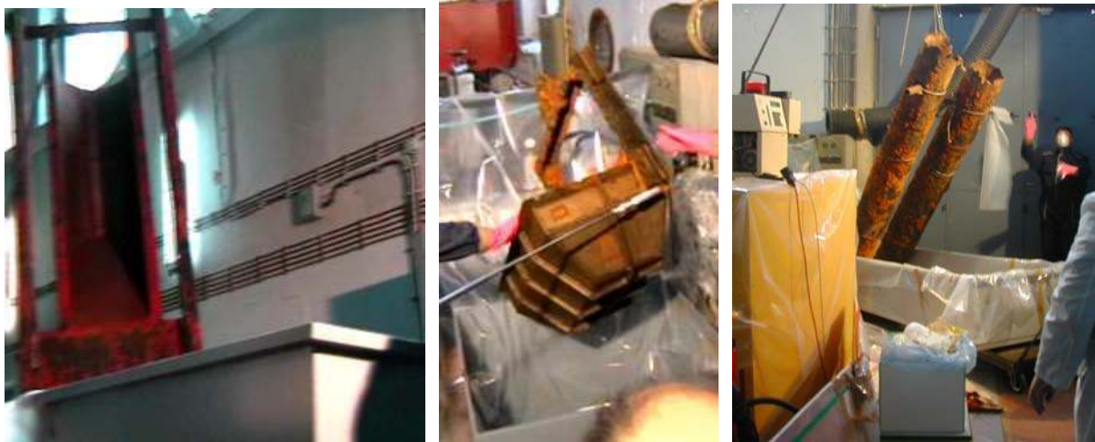
Fig. 2 Removal of the biggest part of metal construction, 'working table' and two inner tubes
