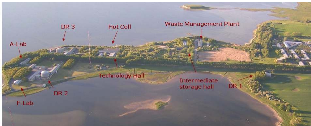
FIG. 1. Location of the nuclear facilities at Risø.
