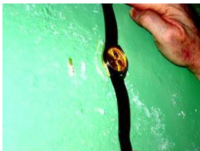
Fig. 1. \text{CaCO}_3 forming on the outer surface of the reactor block near the service pool
