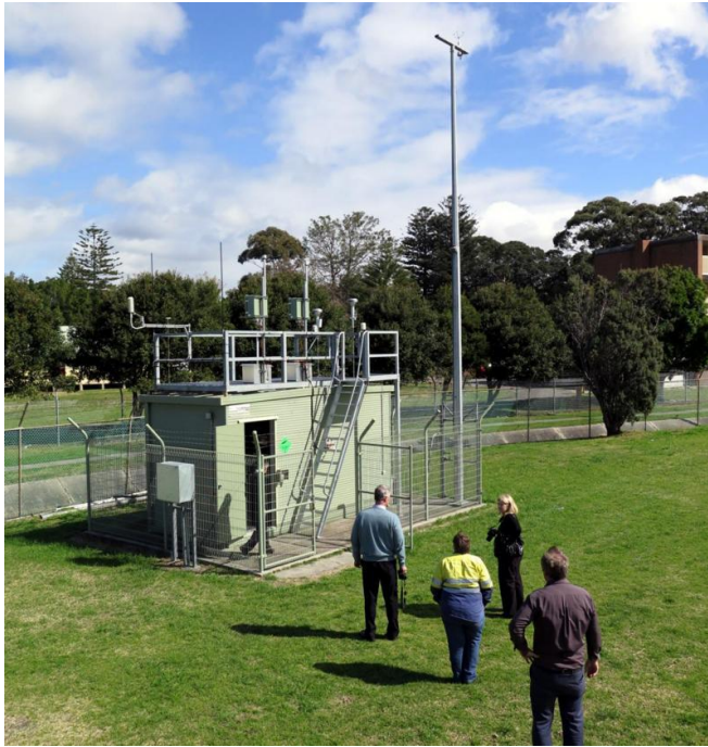
Figure 7: Newcastle Air Quality Monitoring Station during the site visit from the project team
