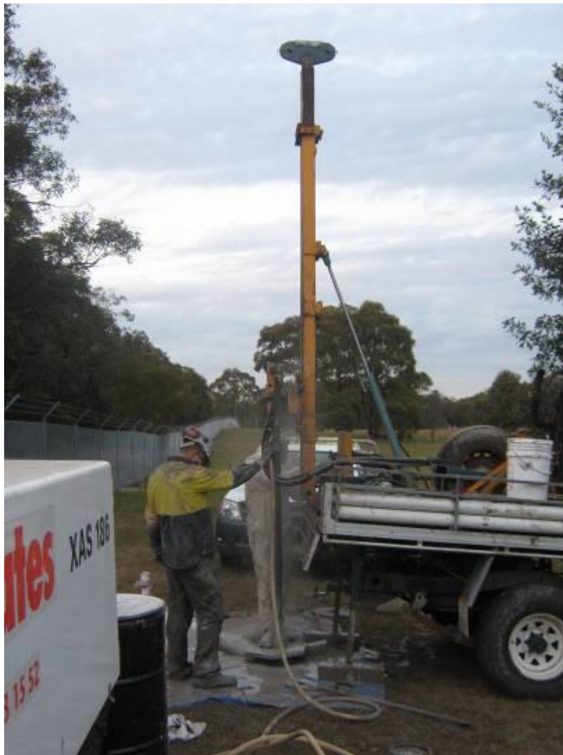
Figure 29. Air hammer drilling at W2D using the Edson MRA260.
