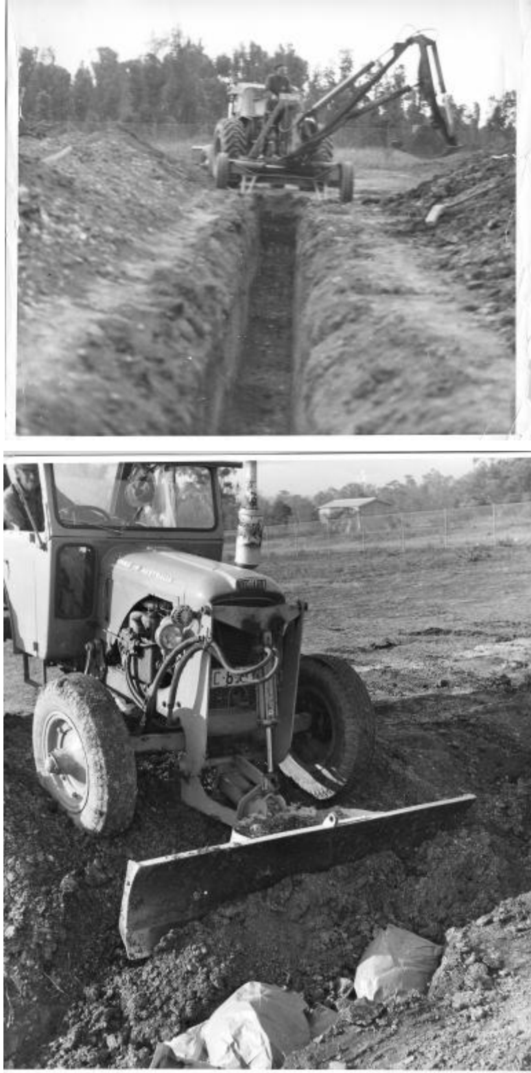
Figure 2. Original a) excavation and b) filling of trenches.
