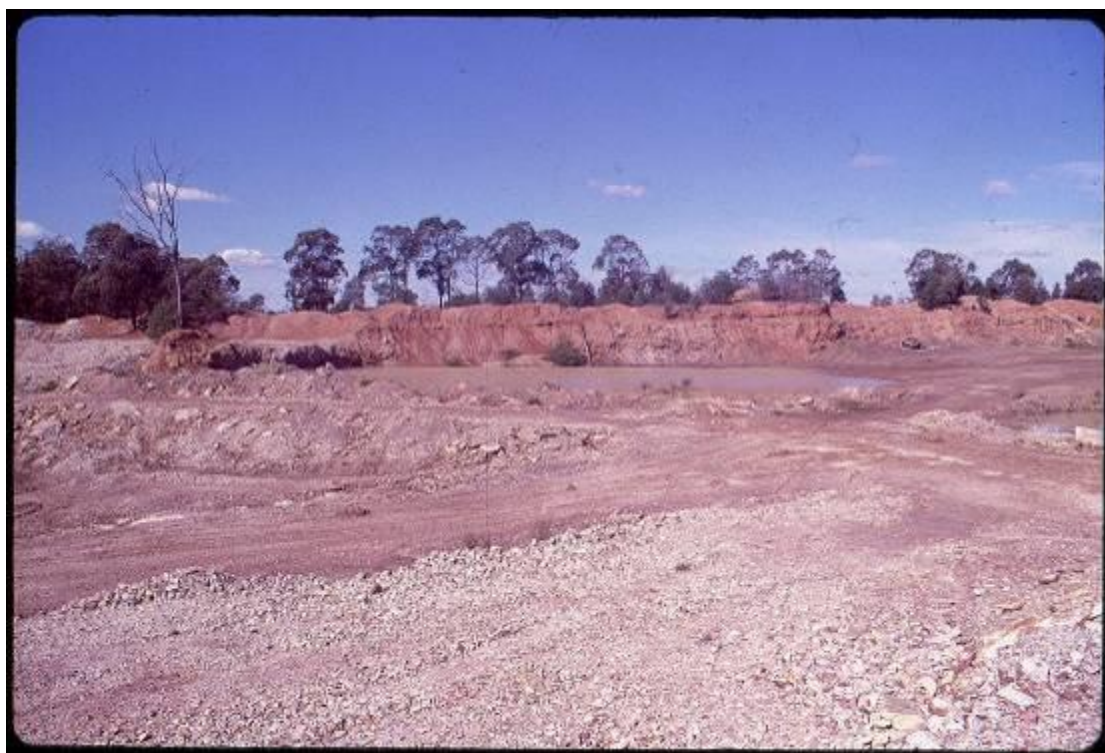
Figure 8. View across Harringtons Quarry prior to remediation, looking east toward LFBG, circa 1984.
