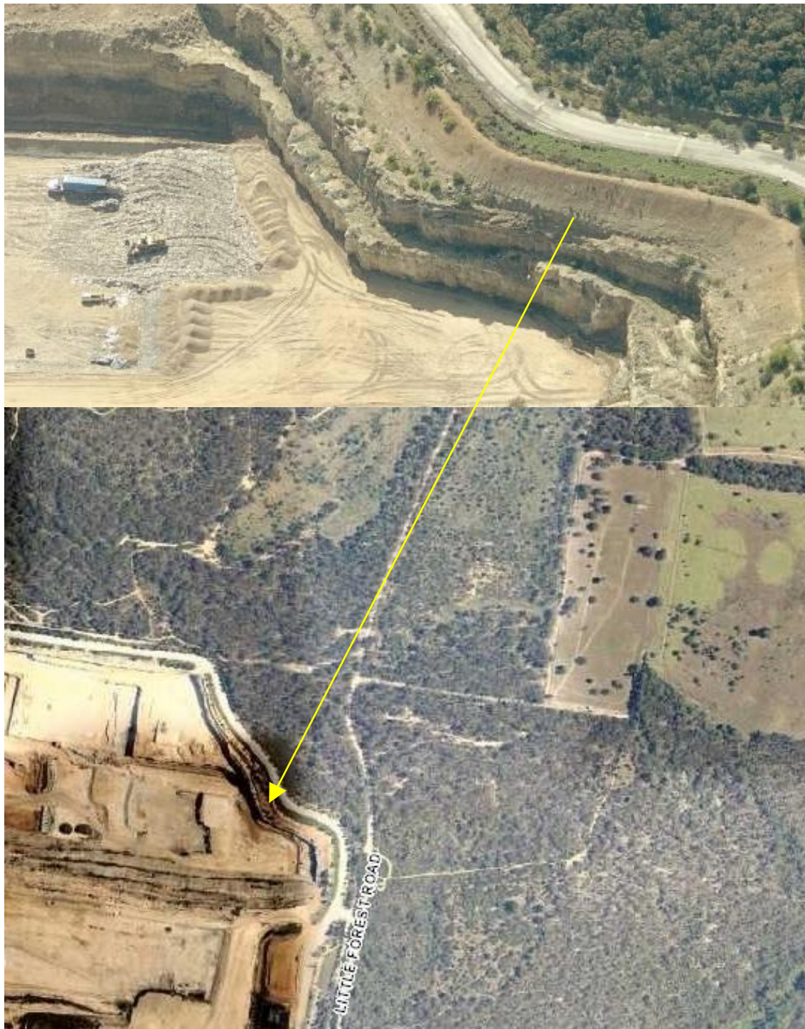
Figure 11. 25-30 m deep face cut in sandstone at Lucas Heights II landfill, 380 m from LFBG, 2012.
