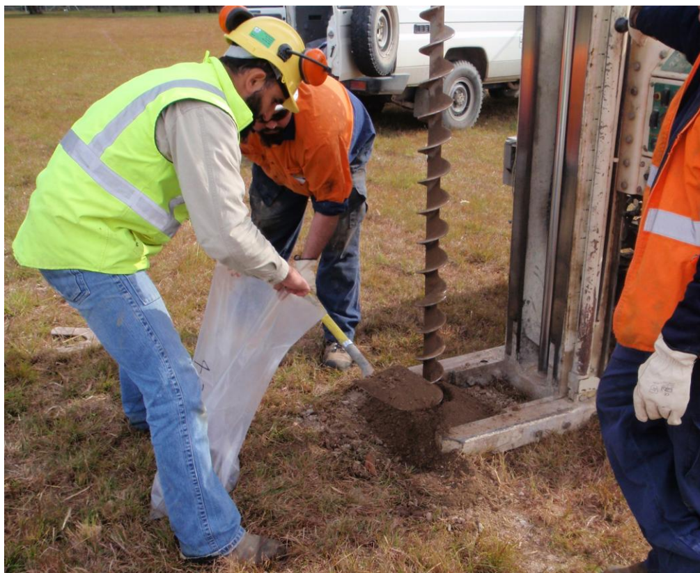
Figure 27. Sampling at CH21 from SFA using the Geoprobe 7720DT.
