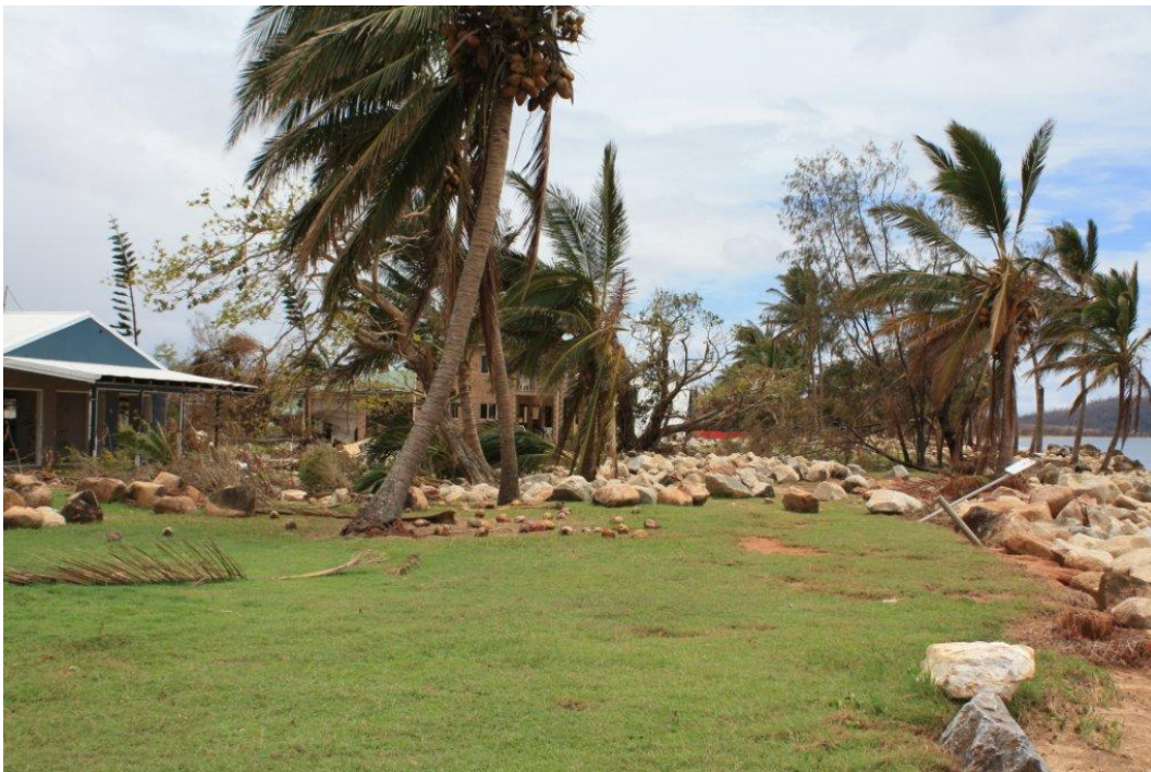
Figure 6: Tully Heads – Looking north towards the boulder deposit sourced from adjacent seawall.
