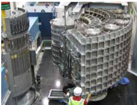
Pelican's massive seven tonne vessel being positioned.
