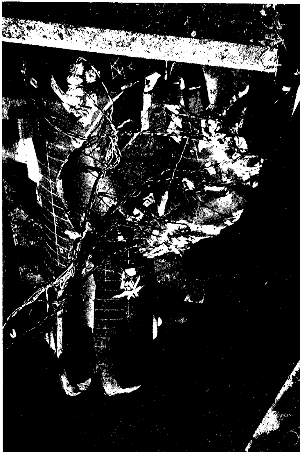
Figure 11 Photograph of failed vessel after removal of bunker roof.
