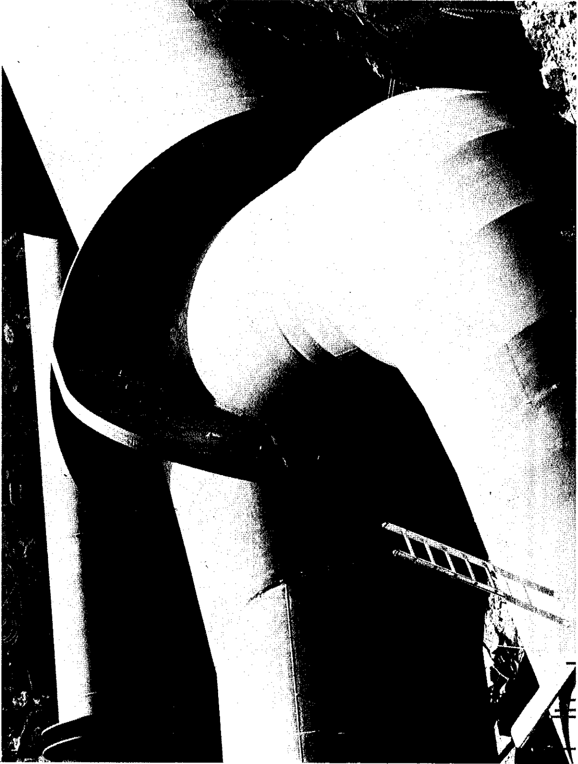
FIGURE 2. BIFURCATE D9. VIEW FROM ABOVE SHOWING REINFORCING RING GIRDERS
