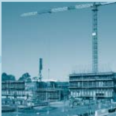
The replacement research reactor under construction.
