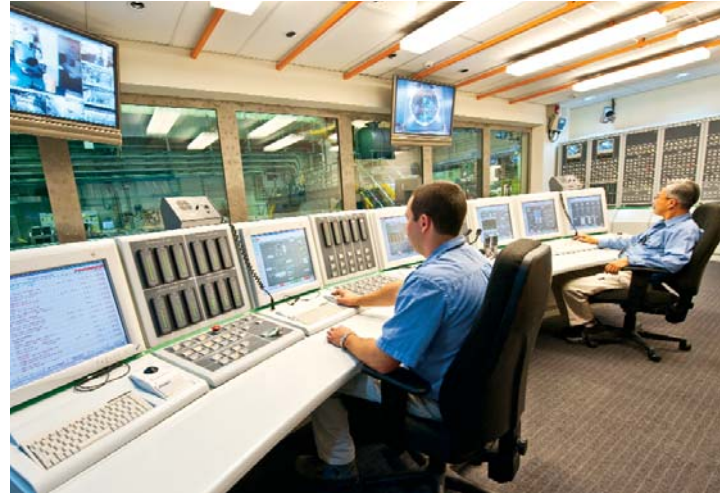
The OPAL control room is where operators monitor the reactor system.
