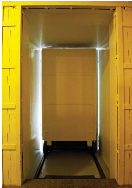
Items are irradiated inside a room with thick concrete walls and door.
