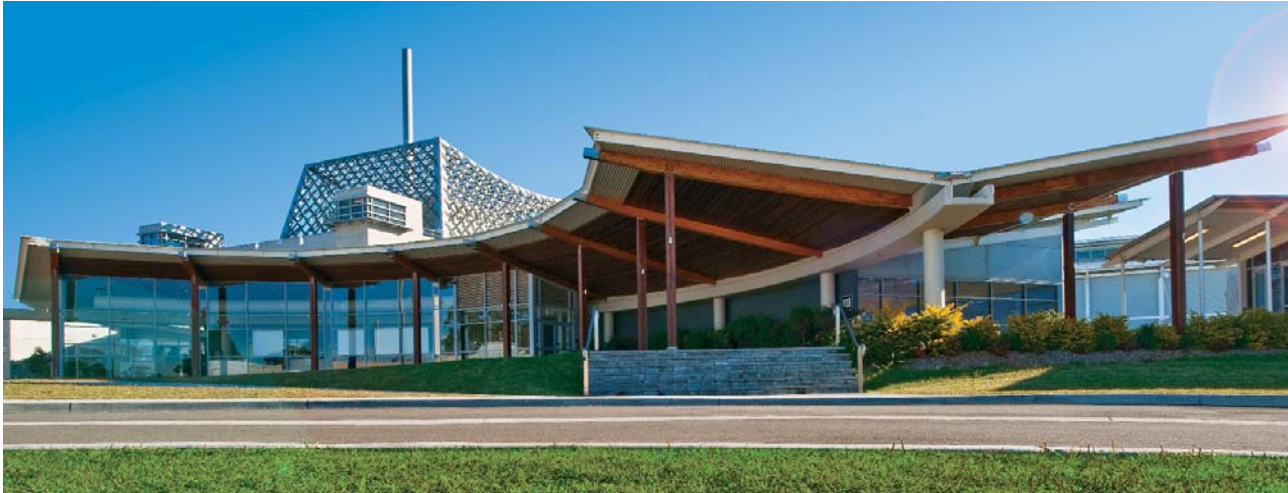
The OPAL reactor building is made from reinforced concrete and has a steel mesh cover which together protect the reactor from external events such as earthquakes and aircraft collisions.
