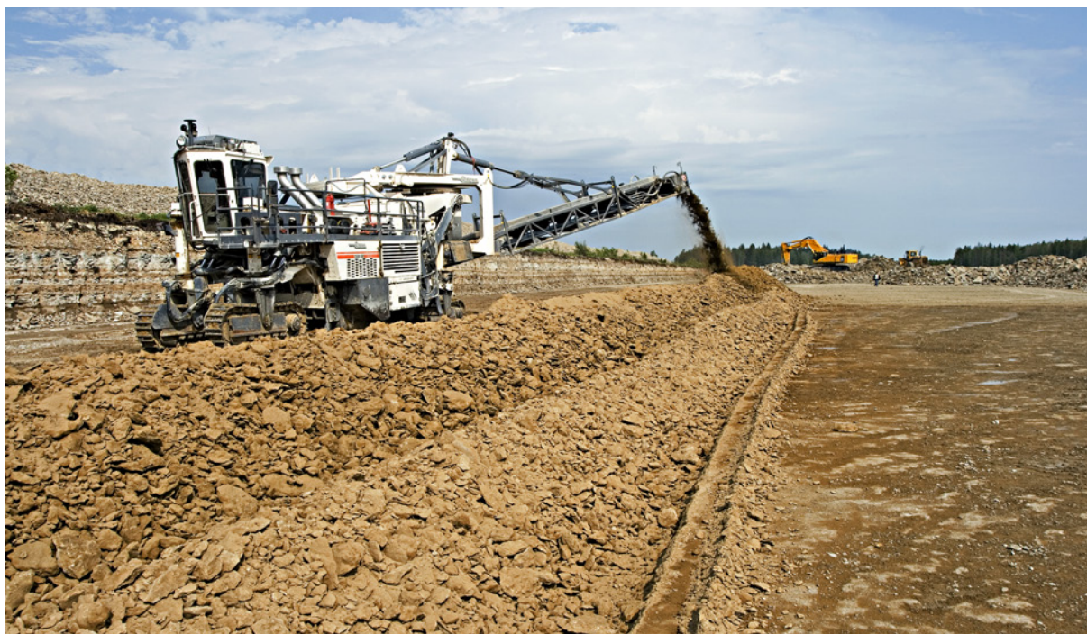
Figure 18. Oil shale mining in the Põhja-Kiviõli open-cast pit, Ida-Viru County. (Photo: H. Bauert).
