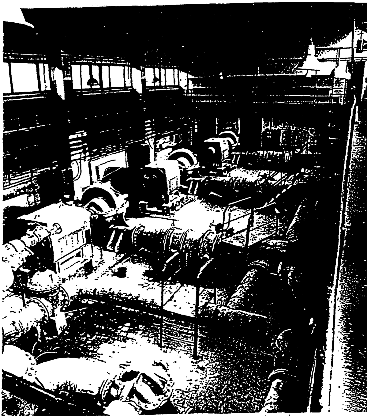
Fig. 19. Reactor equipment in third circuit water circulation pumping block.
