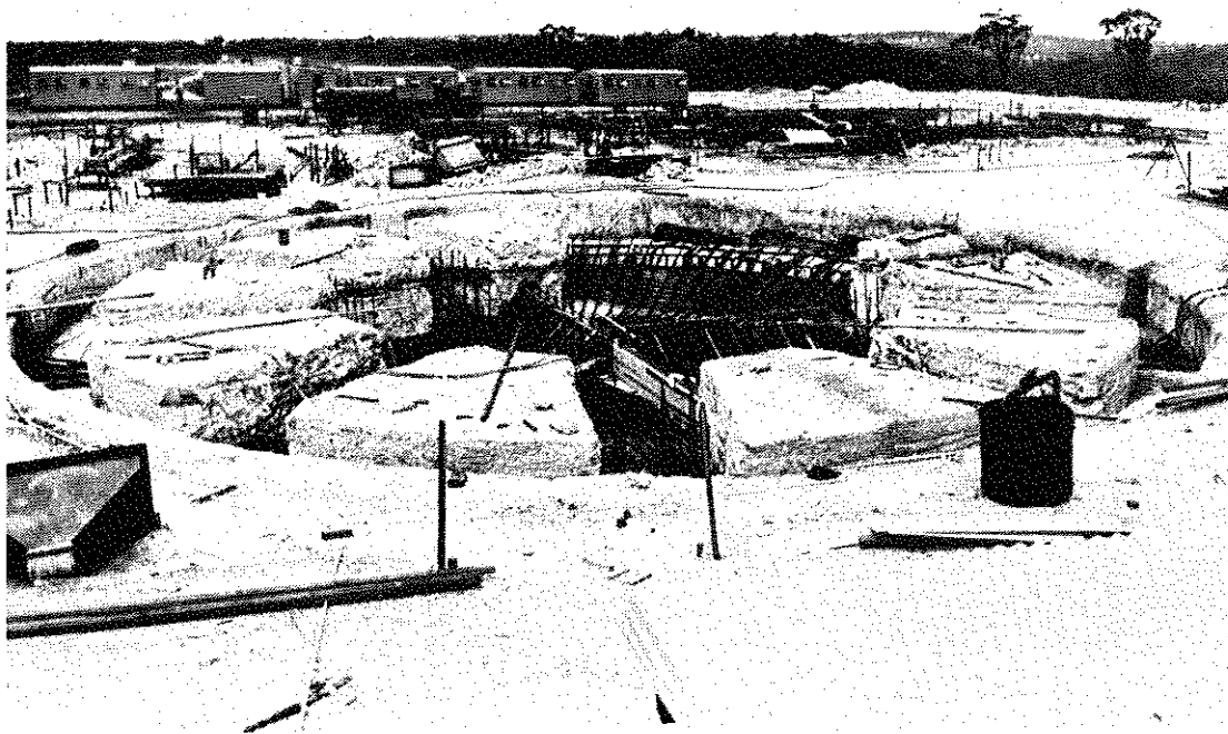
Foundations for HIFAR reactor which were commenced early in 1956.
