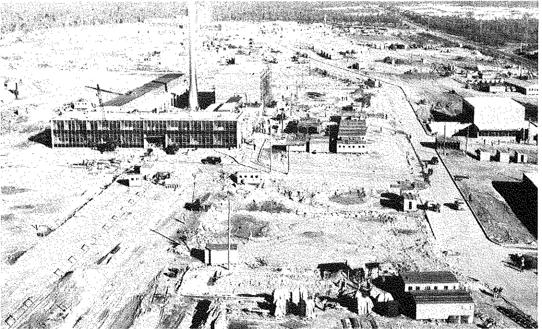
The Chemistry and Chemical Engineering Buildings during construction in 1957.
